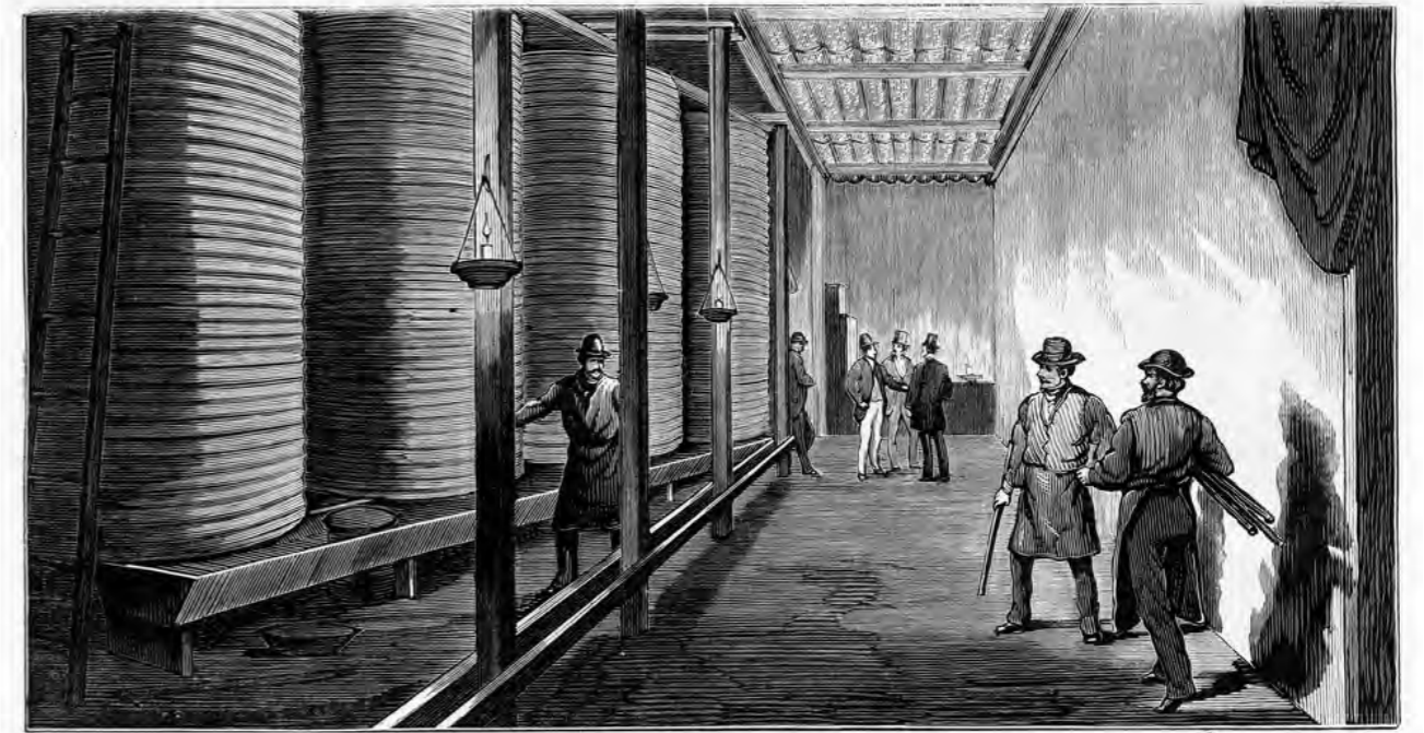
MESSRS. MORT AND CO.'S MEAT PRESERVING WORKS, DARLING HARBOR, SYDNEY. 1.—THE ICE MAKING ROOM. 2.—THE COOL OR FREEZING ROOM. 3.—MILK PRESERVING ROOM.
